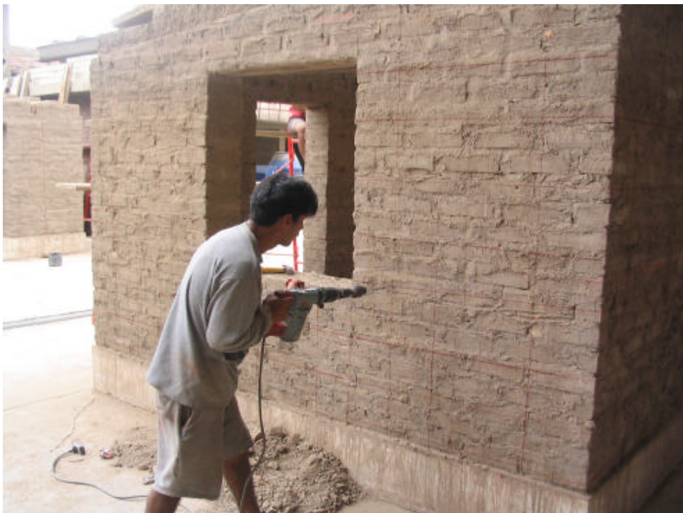
Figure 7. Drilling holes in the wall, spaced every 30 cm.
