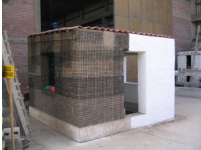
Figure 14. Model 2, reinforced with polymer geogrid and plastered for one side.
