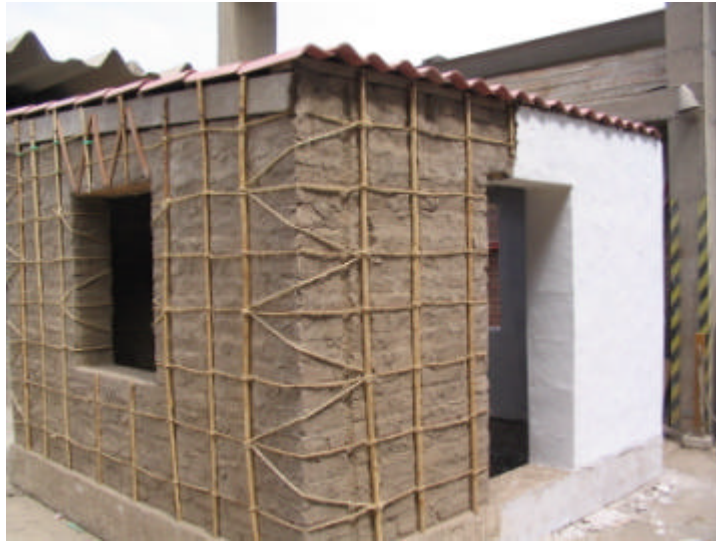
Figure 6. Model 1 reinforced with natural materials and plastered on one side.
