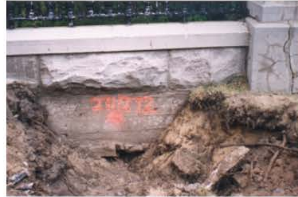
Foundation excavation at 1933 Section
