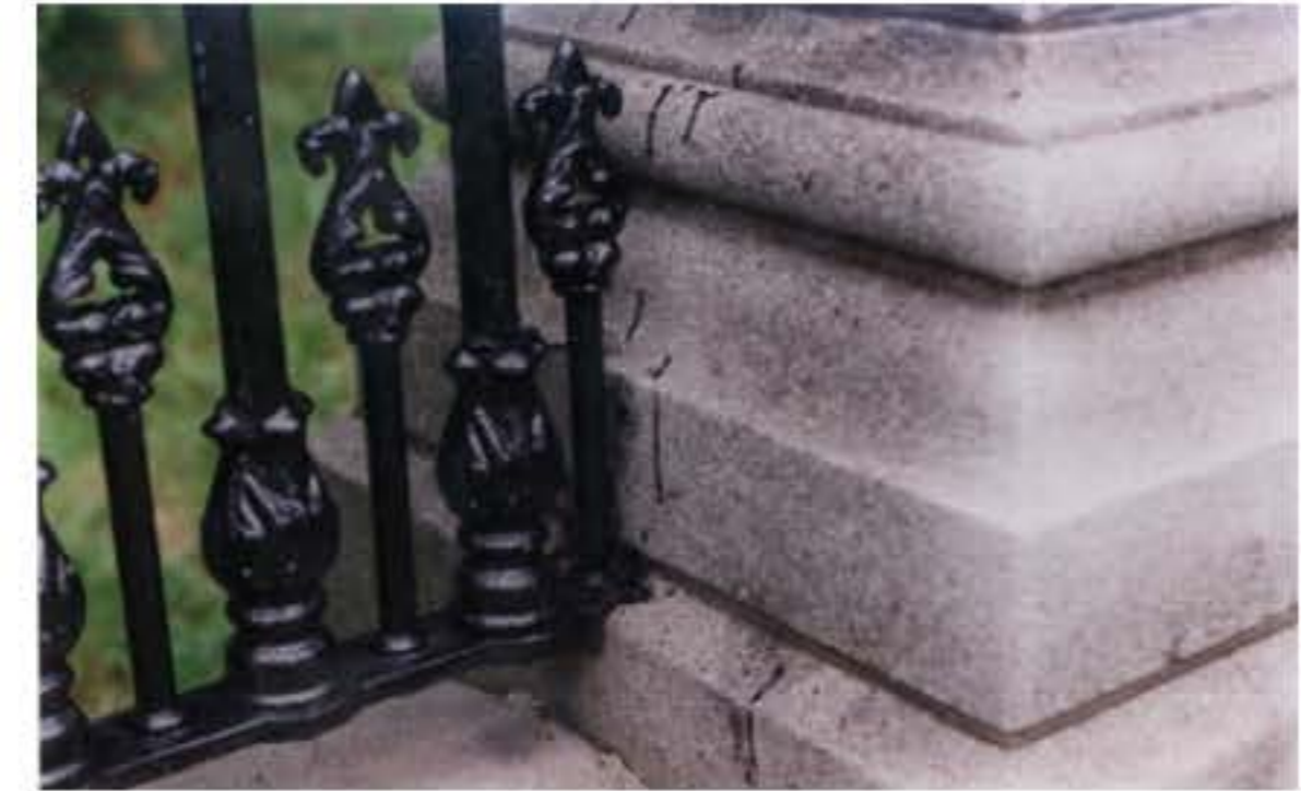
Routine maintenance is required for paint touch-ups, and cleaning of masonry
