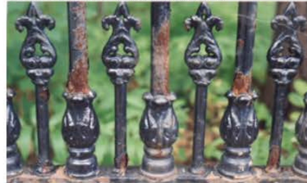
Typical deteriorated metal work, 1933 Section
