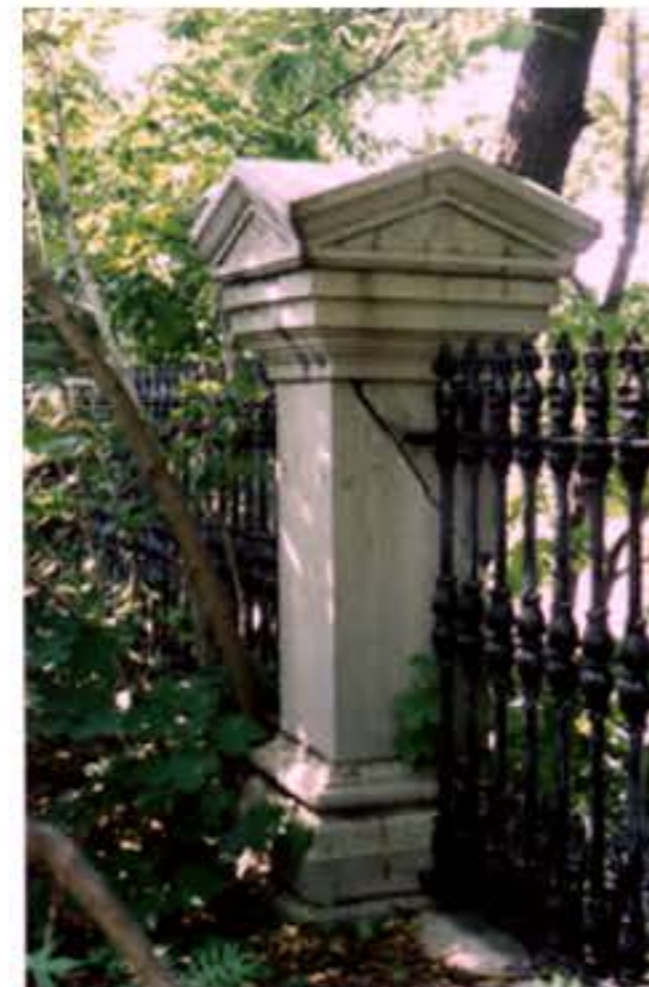
Overgrown vegetation at 1939 Section
